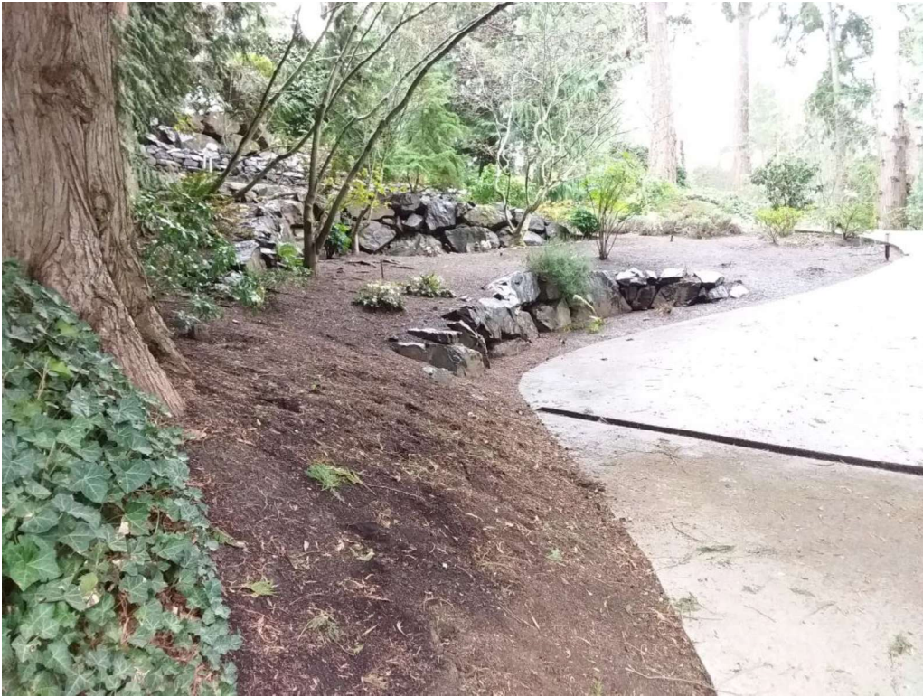
Figure 12. Looking SSE at the driveway curve and stone walls on the south side of the #7 Leyland cypress.
