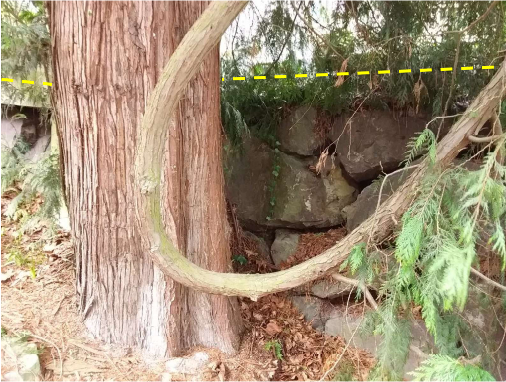
Figure 5. Looking SE at the base of the #2 cedar. Note the level of the parking slab for the 4651 house.
