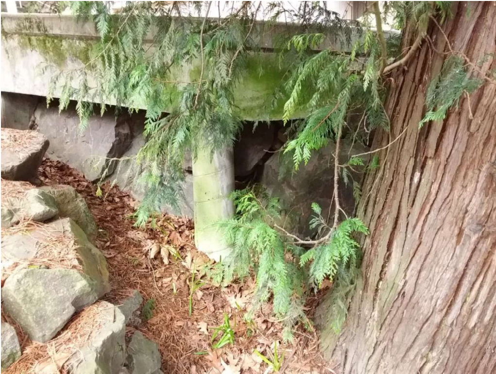
Figure 6. Concrete support post for the 4651 parking area.
